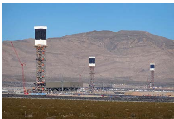
Three Power Towers in the Ivanpah Plant
